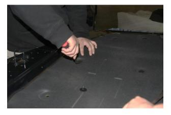
**Step 6:** Place the heat shield over your carbon hood- this will give you an idea if minor adjustments may be necessary. In this case we used a dremel to cut along the sides of the indentations that were on the carbon hood. Be careful when cutting so you do not cut through the hood.
